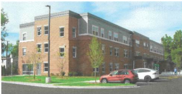
View from the SE corner
